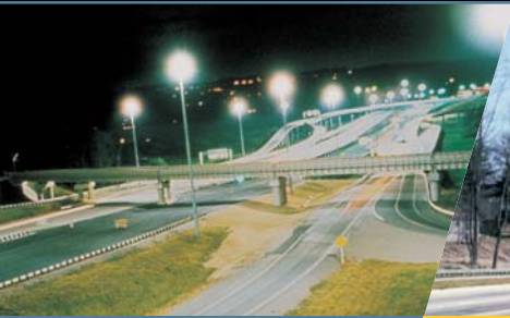
High Mast Lighting
