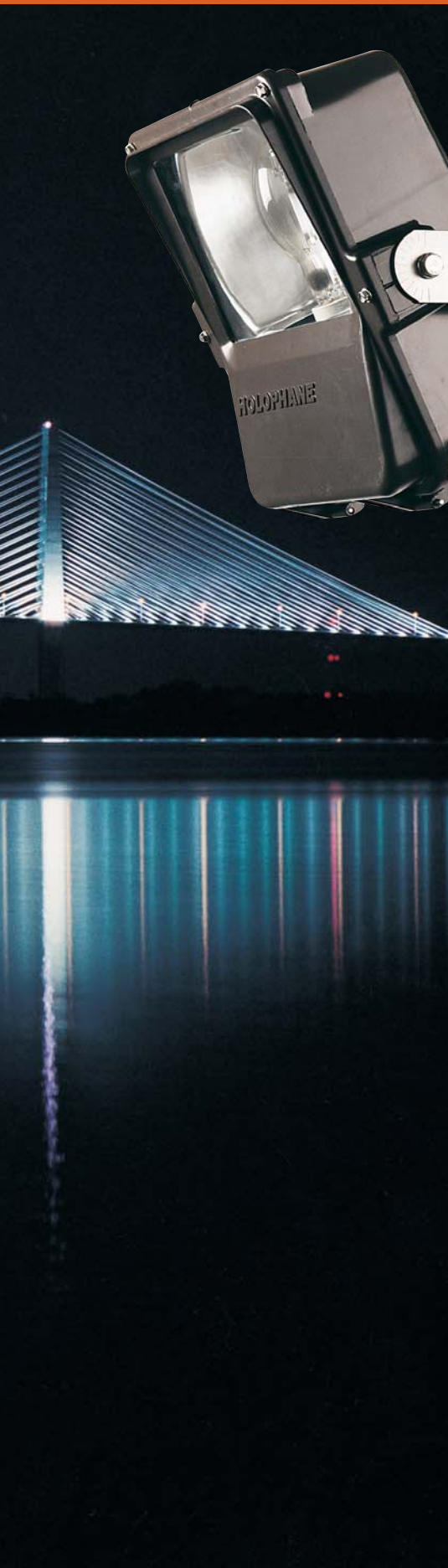
Dames Point Bridge, Jacksonville, Florida
